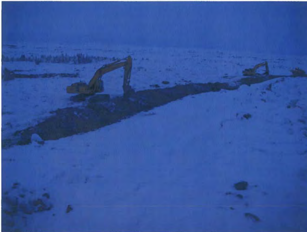
FIGURE 6: DIVERSION DITCH – LOOKING NORTHWEST
