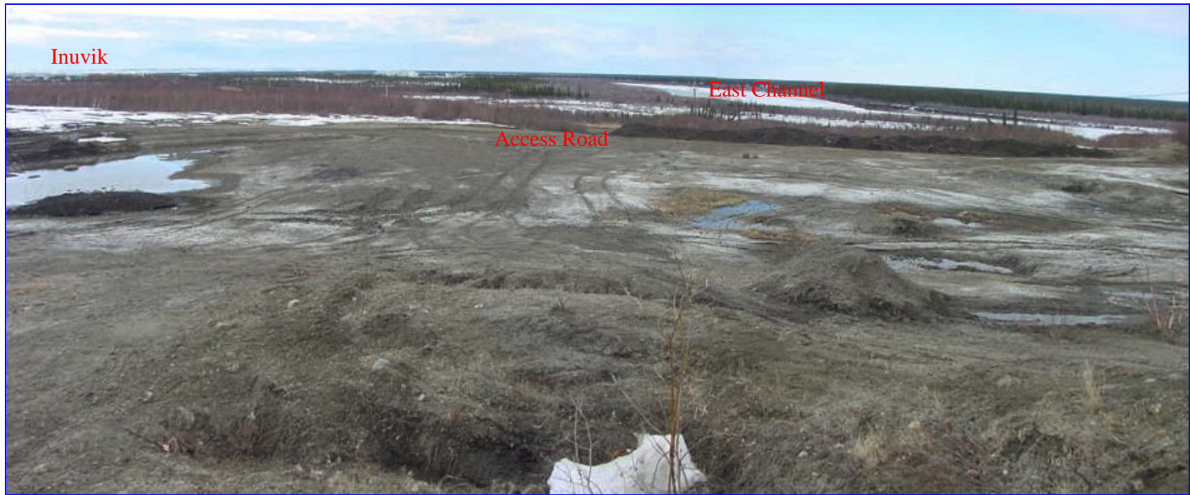
Photo 1: Looking southeast at the abandoned pit north of Inuvik, where Aurora College (Aurora Campus) proposes to erect a Rig Training Facility. The abandoned pit runs adjacent to Navy Road with three access roads. May 31, 2001.
