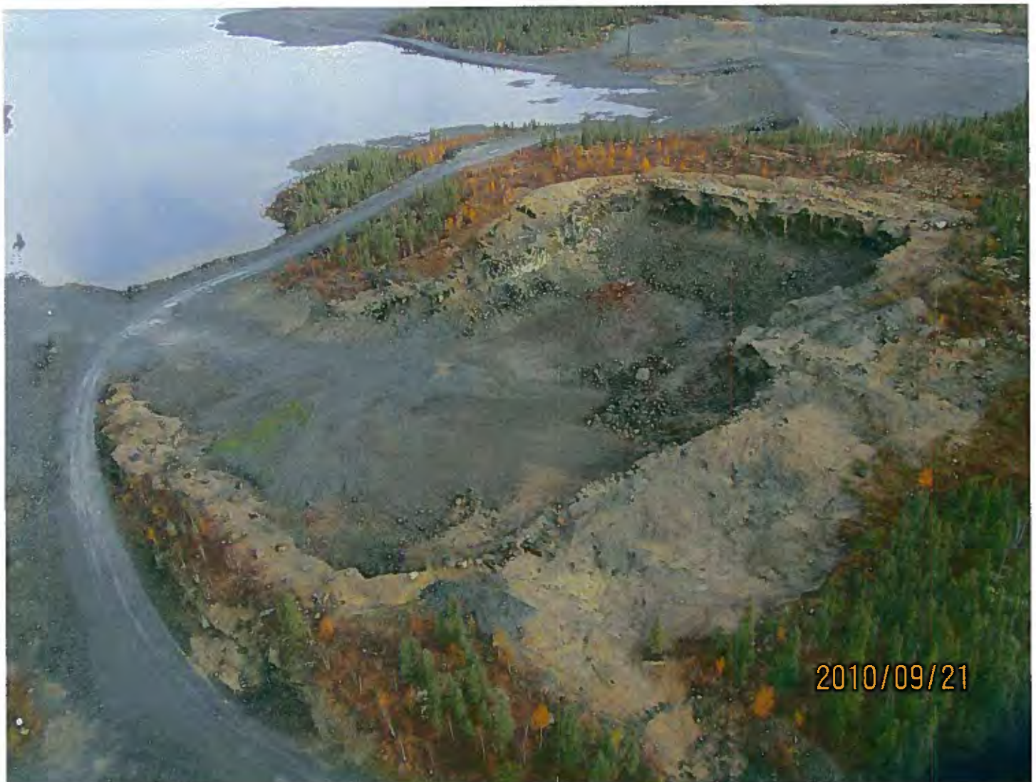
W2009X0007 - Colomac Mine Site - INAC-CARD Tailing quarry and oversized rock in the centre of the quarry must be tucked up against the working face.
