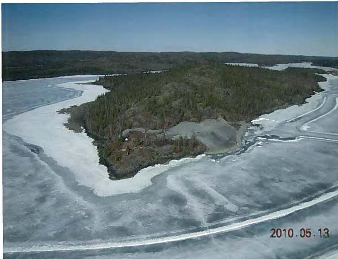
W2009X0002 - North Inca - Indin Lake Looking north at the land use area where the mine infrastructure has been removed and the camp was set up.
