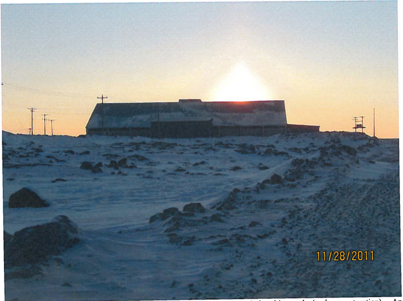
Figure 3. AN storage building as viewed from one of the new wind turbine pads (under construction). An inspection of the building showed no environmental concerns (it was being operated as per best practices, with AN stored below the height of the cement walls).
