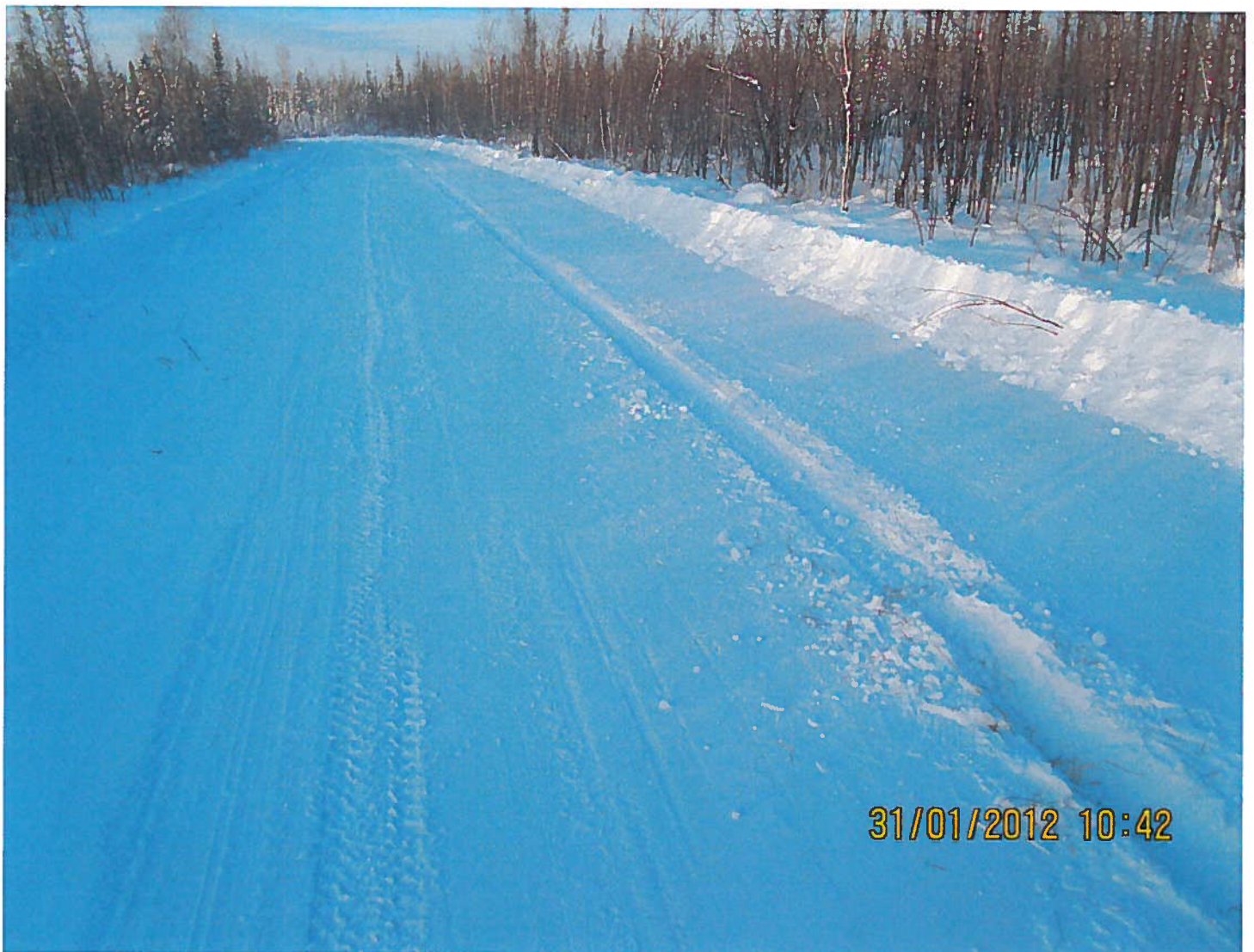
W2007F0001 - NTPC - Winter Road - Km 4 of the Wekweeti Road to Snare Forks. Photo #3 - Rutts made by a pickup during the inspection.
